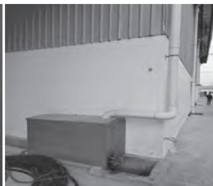
Rainwater harvesting tank
