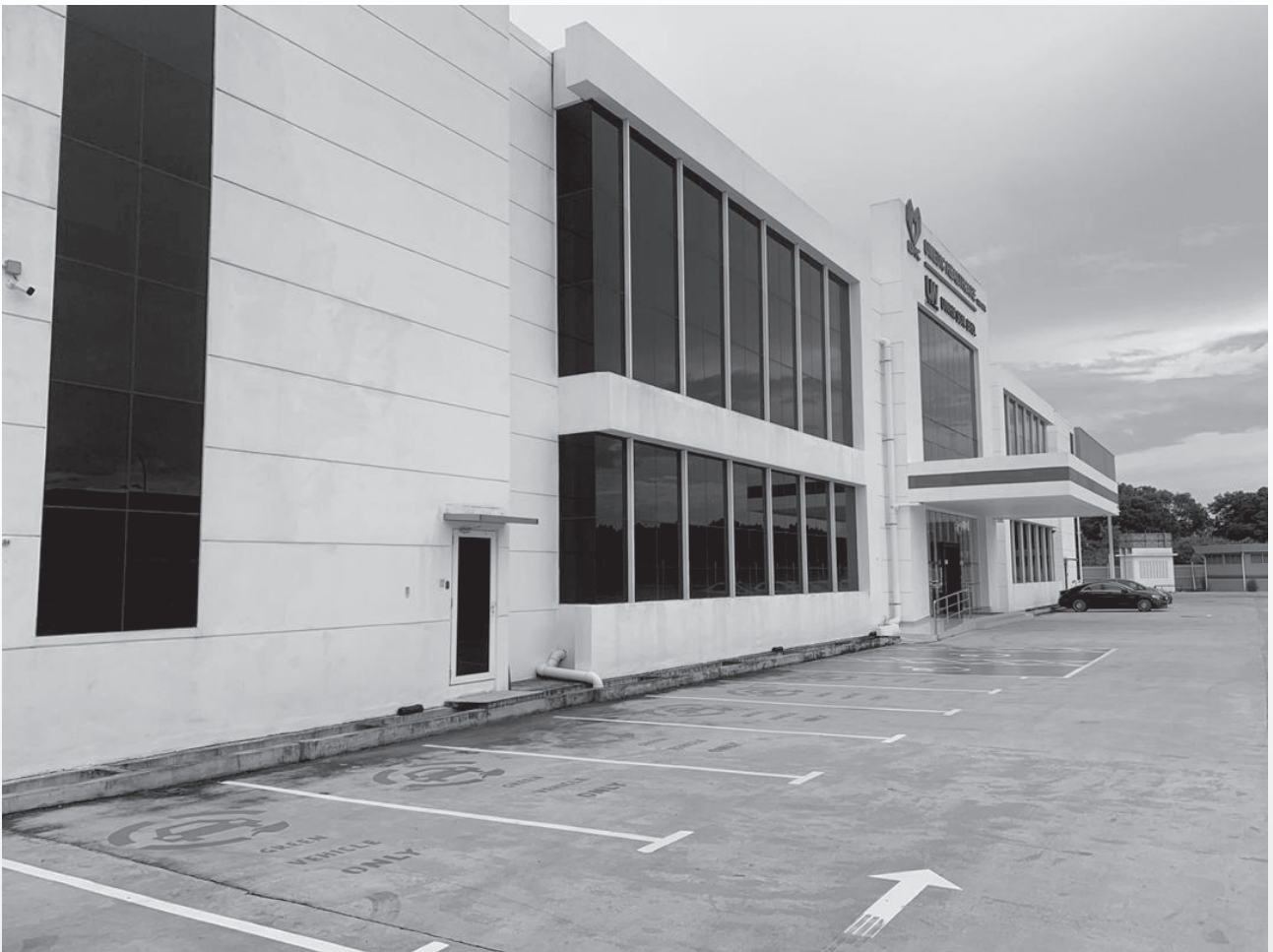
Designated parking space for green vehicles
